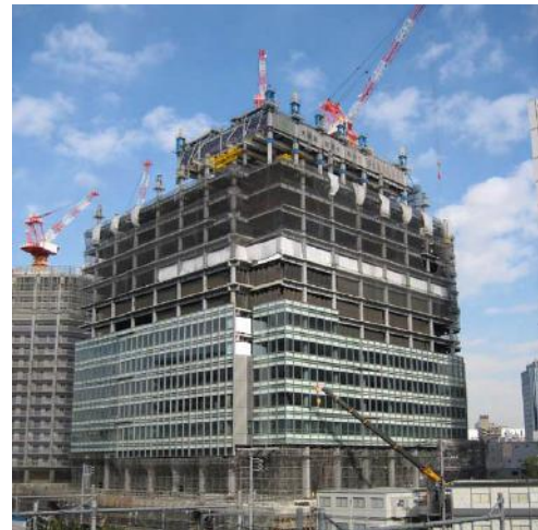
Photo 2. Building of Project O under Construction
