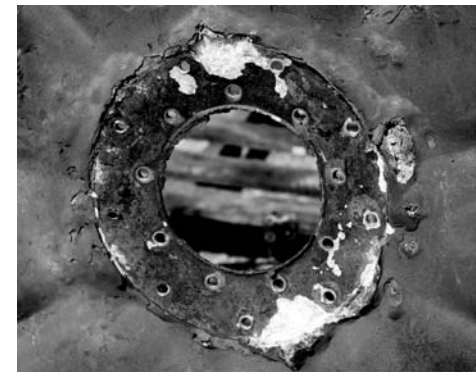
Fig. 7 Firing platform exfoliation corrosion. Source: Ref 5
